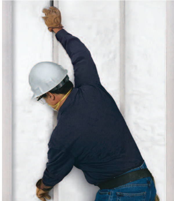
Acoustical insulation being installed in interior wall cavities.
