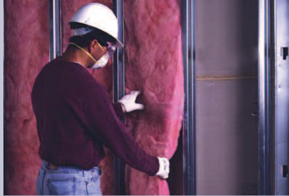
Acoustical fiber glass batts and duct insulation are known for their excellent sound control properties.
