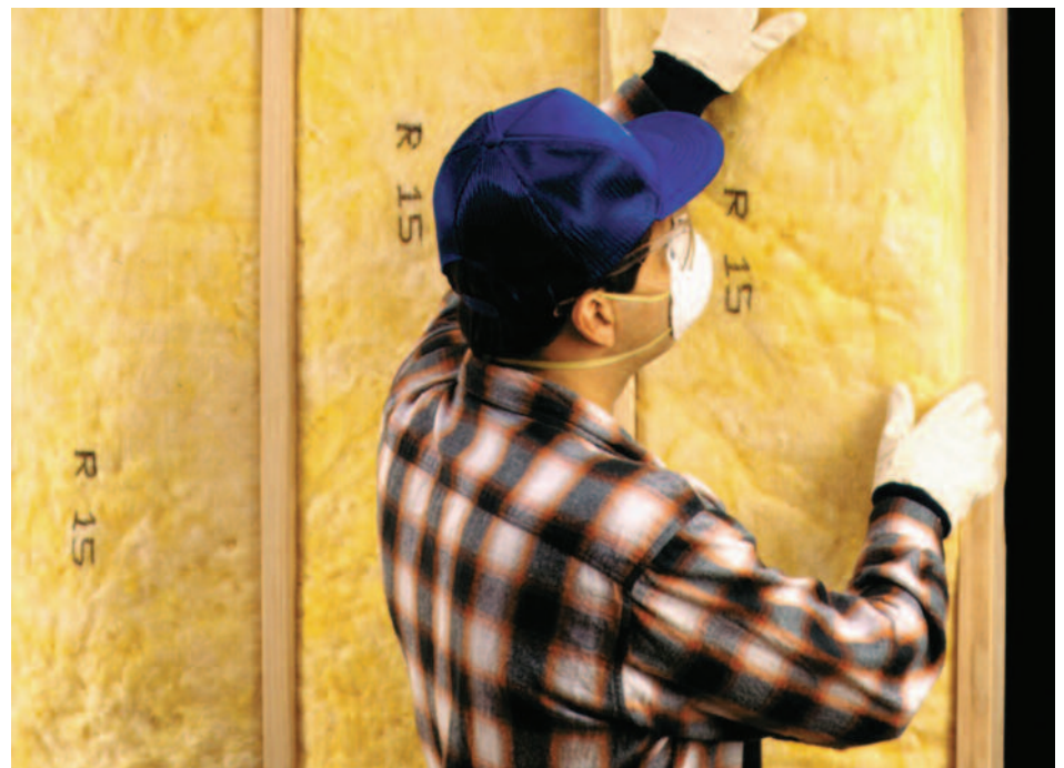
Fiber glass acoustic insulation being installed in an exterior wall.
