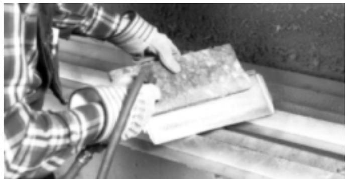
*Fig. III-3. Applying duct liner adhesive with spray equipment. Adhesive may also be applied with brush or roller.*
