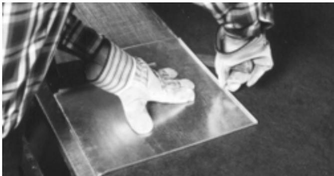
*Fig. II-1. Cutting fibrous glass duct liner by hand.*
